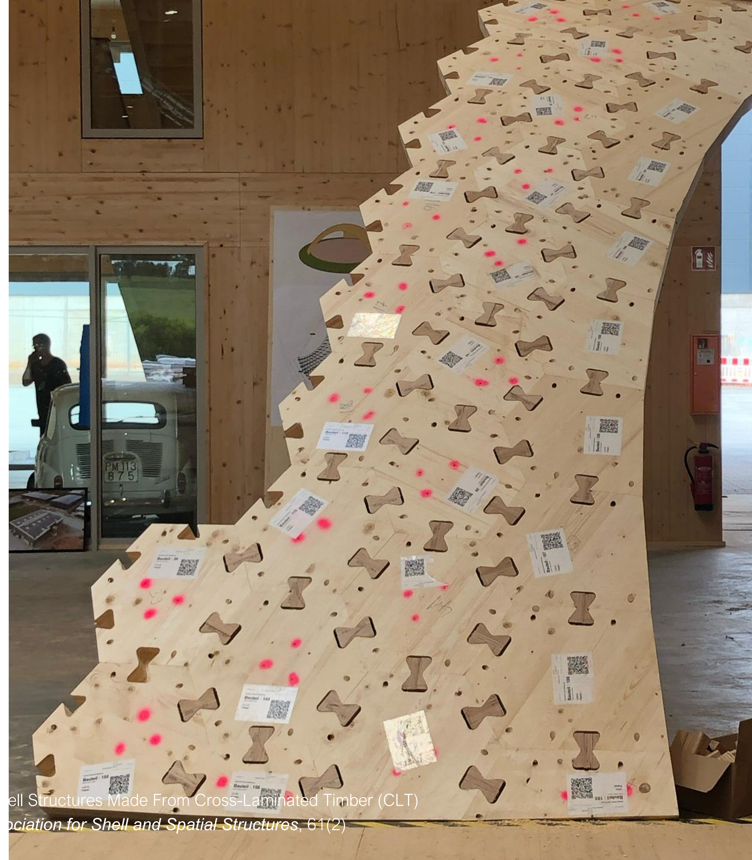
Robeller, C., Von Haack, N. (2020), Recycleshell: Wood-on-Shell Structures Made From Cross-Laminated Timber (CLT) Production Waste, in Journal of the International Association for Shell and Spatial Structures , 61(2)
