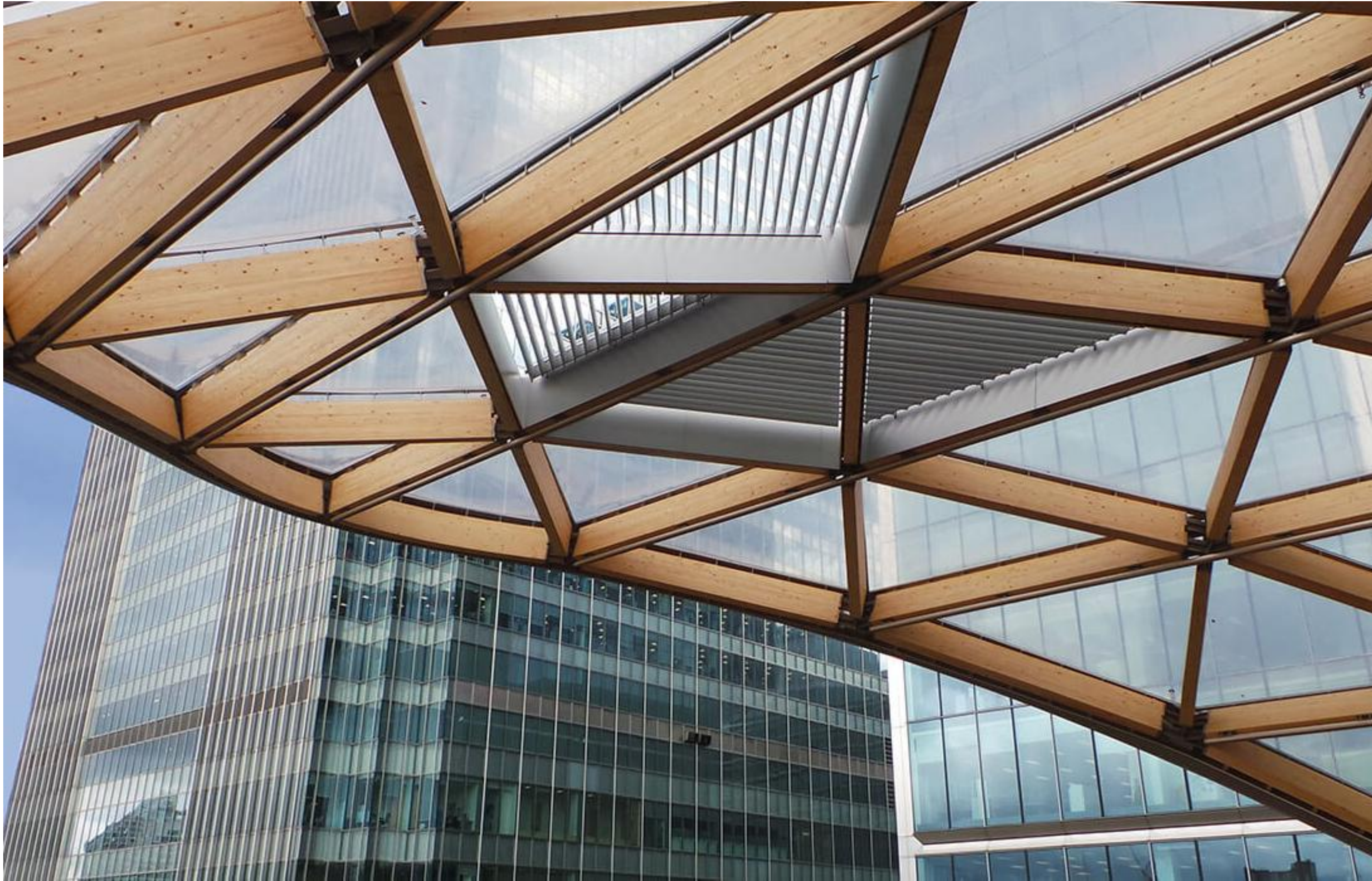
Crossrail Station 2014, Foster and Partners, London
