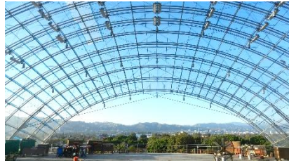
Academy Museum of Motion Pictures, Los Angeles, 2021 Renzo Piano Building Workshop, Genoa
